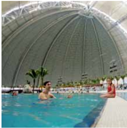
Tropical Islands Resort near Berlin, Germany A steady 25° C air temperature, 31° C water temperature, no rain, and a pleasant 40% to 60% humidity for the resort's tropical plants. Everyone's idea of perfect weather! All this is possible with a first class climate and water control system driven by VLT® HVAC Drives.
