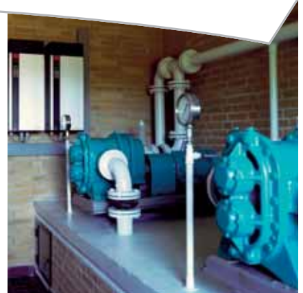
Flexible compressor mode operation even above nominal speed and high break away torque for start-ups allow for better control and major savings.
