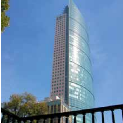
Torre Mayor, Mexico City With its 55 floors and a height of 225 m the Torre Mayor is the highest building in Latin America. Danfoss drives control the heating and ventilation.
